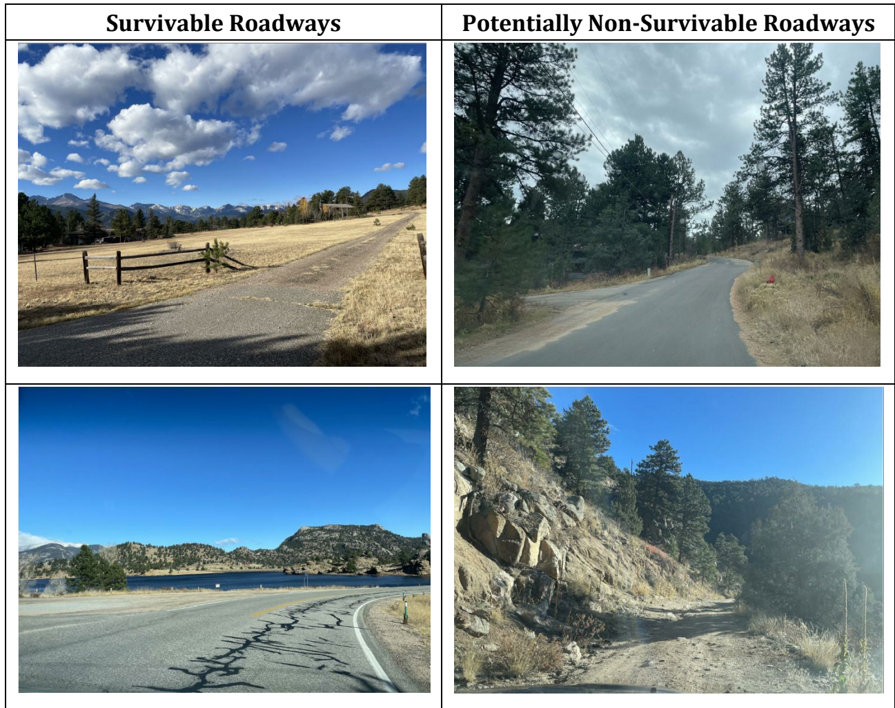
Figure 8.a.11. Some roads in the Estes Valley Fire Protection District have been well mitigated by removing tall trees and saplings, removing limbs on the remaining trees, and keeping grass mowed (left images). Other roads could experience potentially non-survivable conditions because they are lined by thick forests that have an abundance of ladder fuels (right images). Photo credits: The Ember Alliance.
